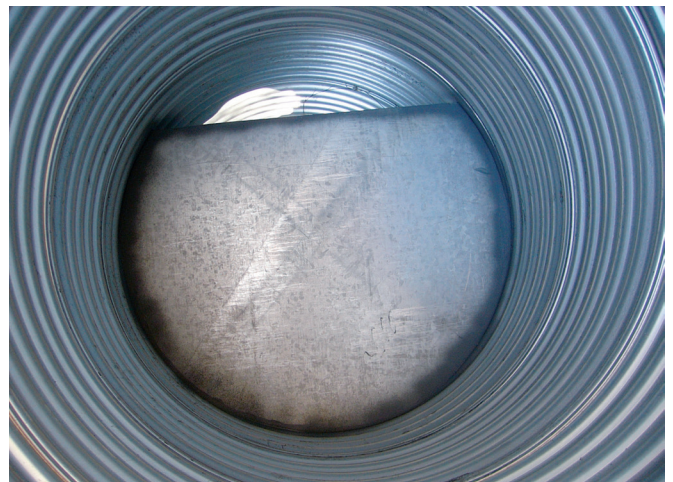
Clapet anti-retour
